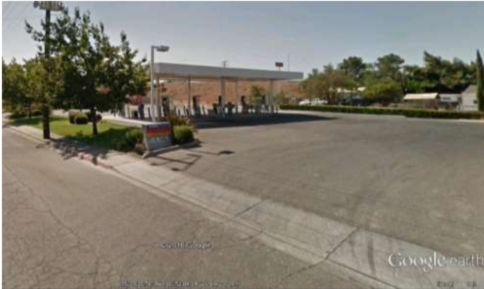
Figure 3-2 Unmanned Pacific Pride “Card Lock” fueling Site
