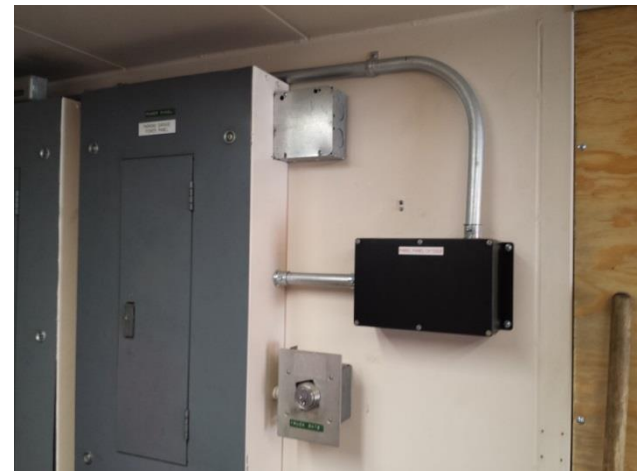
Typical Installation near Breaker panel
