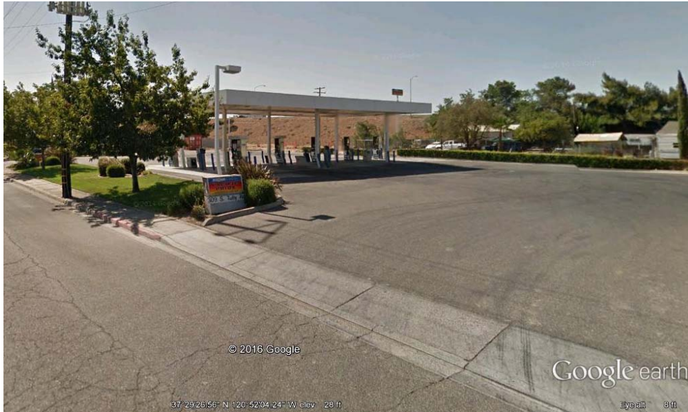
Figure 9.2 Unmanned Pacific Pride “Card Lock” Fueling Site
